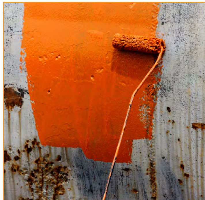
Protection against corrosion
