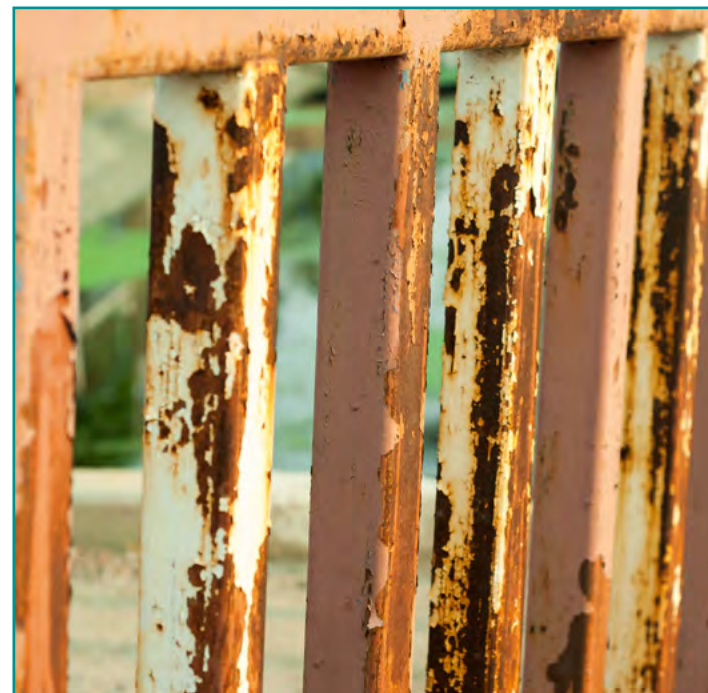
Fench corrosion
