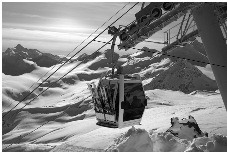
metal wire to support the cable car
