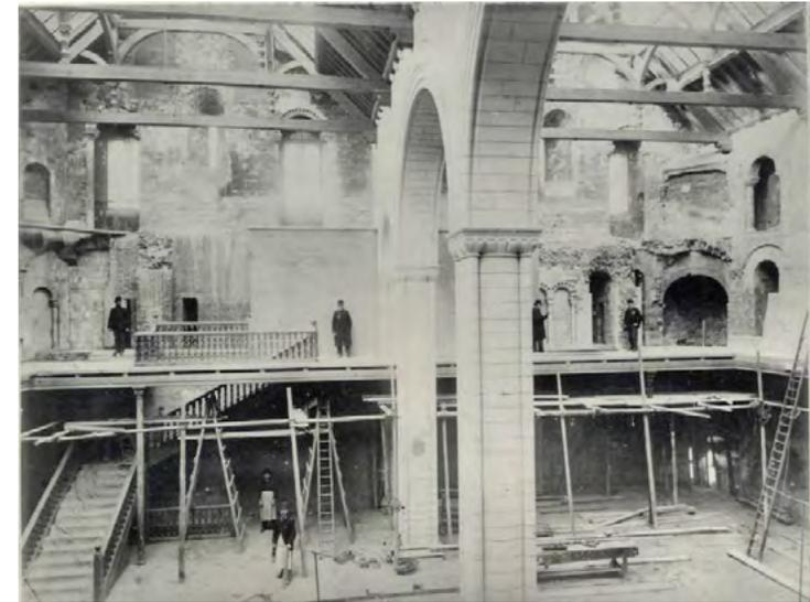
Modern arches, designed to look Norman like the Keep, were inserted to hold up the new roof, and a wooden walkway inserted around the edge
